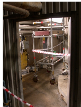
Temporary barrier for high-pressure spraying, soda recovery unit 4
